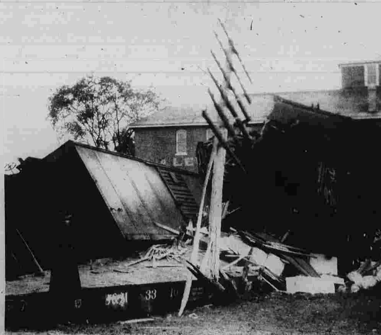
Wreck of the Bullet The Bullet, an express freight train headed from East Hartford, jumped a switch at Apol's Crossing Oct. 23, 1933, causing a train wreck that was long remembered. Every car derailed and telegraph poles were snapped off like matchsticks, but no one was seriously injured. (Fallot photo)
