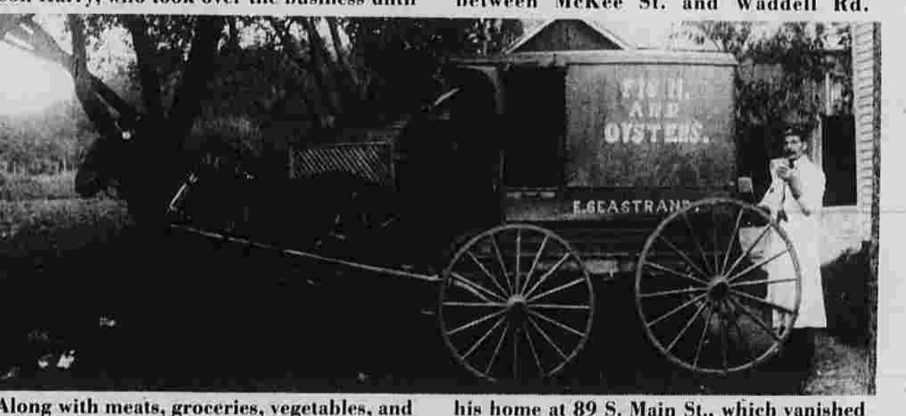
Along with meats, groceries, vegetables, and milk, fish products were sold from house to house in the early years of this century. Emanuel Seastrand's base of operations was his home at 89 S. Main St., which vanished from the scene with the construction of I-84. His sons carried on the business for a number of years from the same location.
