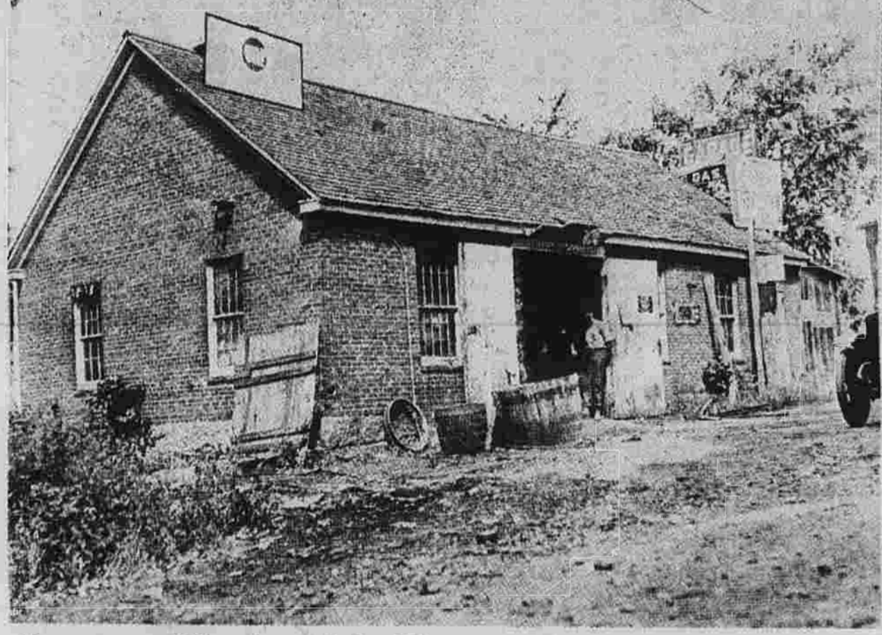
Lyman Blacksmith Shop, Manchester Green
