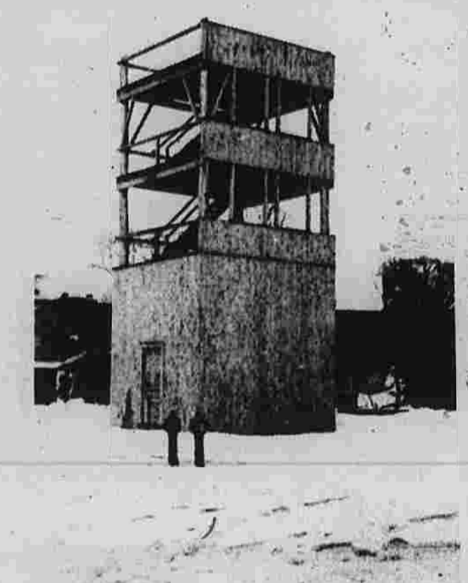
The South Manchester Fire Department's drill tower, off Hartford Rd., was used from its completion Aug. 17, 1917, until Spring of 1959. The tower, once 45 feet high, was built by Cheney Bros. on company-owned land. It eventually began to rot, and on Jan. 13, 1961, it was knocked down and burned.
