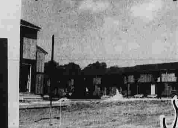
Homestead Park Village CONGRESS AND HOMESTEAD ST. (FIRST PHASE NOW BEING COMPLETED)
