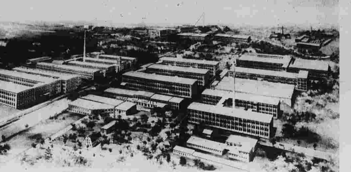
Cheney Bros. Mills in 1923. At left, throwing upholstery and dress goods weaving mills. Front center, spun silk mills, store house, and machine shop. At right, front to back, ribbon mills, velvet weave shed, yarn dye house, and spun silk dressing mill. Total floor space in the complex was 35 1/2 acres.
